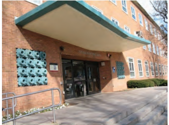
Photo 5-1: View of Fine Arts Building
