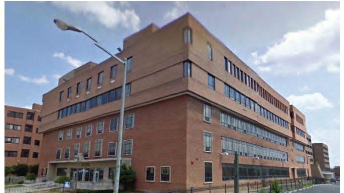
Photo 5-10: View of College of Dentistry Building
