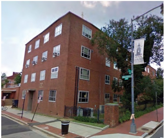
Photo 5-12: View of Chauncey L. Cooper Hall/College of Pharmacy
