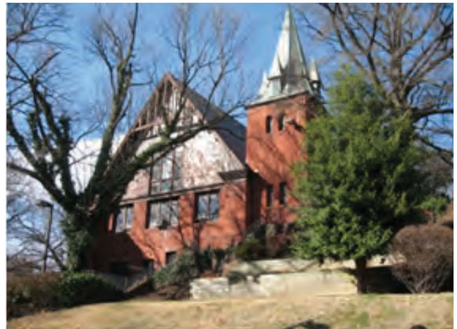
Photo 5-19: View of Rankin Chapel West Elevation
