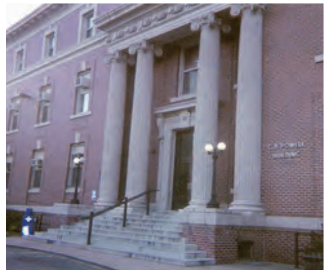
Photo 5-8: View of C.B. Powell Building
